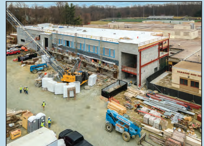
HCPSS School Construction and Renovation
